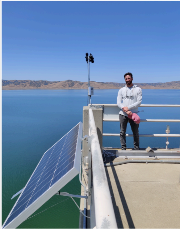
Figure 8. Installation of Gybe sensor at San Luis Reservoir, California by project scientist Adam Belmonte (2021).
